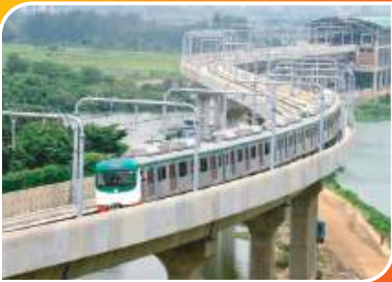
Metro Rail Dhaka
