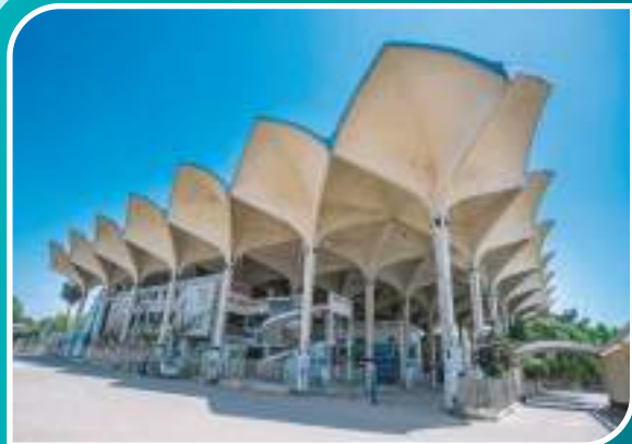
Kamalapur Railway Station, Dhaka
